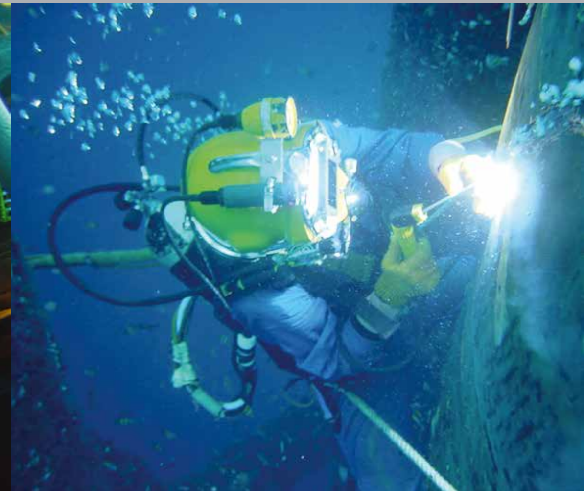
UNDERWATER WELDING FOR SALVAGE OPERATION
