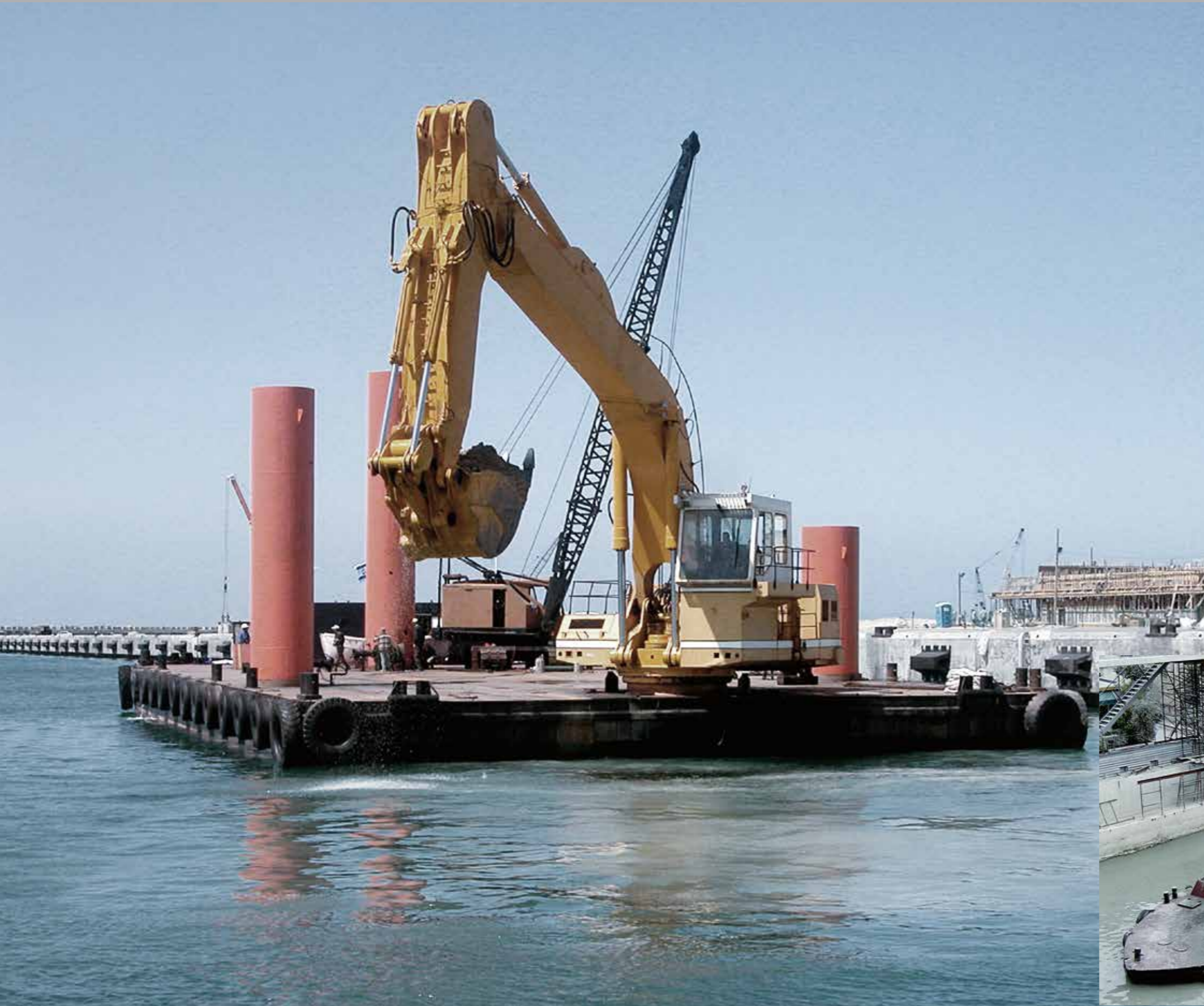
PORT MAINTENANCE EXCAVATION
