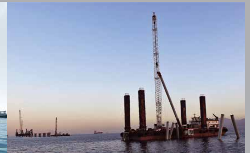
DRIVING OF STEEL PILES
