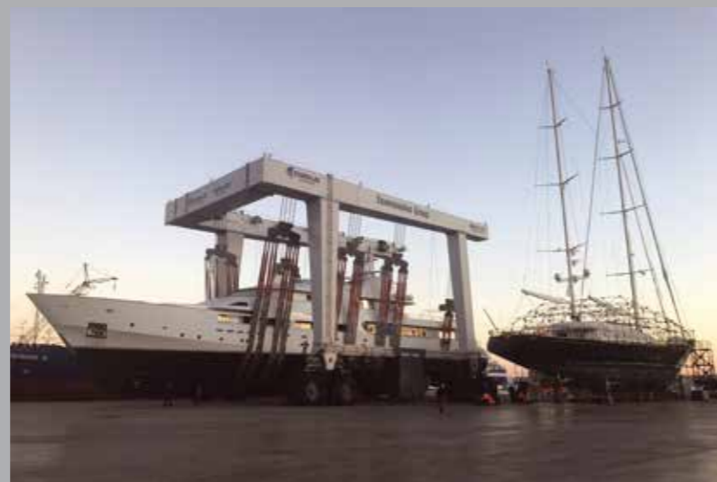
HAULING OF A 55N CRN YACHT & MAINTENANCE WORKS ON A 48M PERINI NAVI
