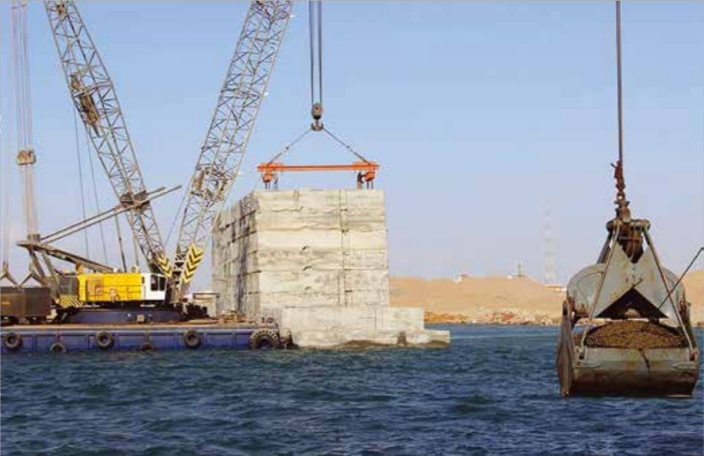
QUAY WALL CONSTRUCTION
