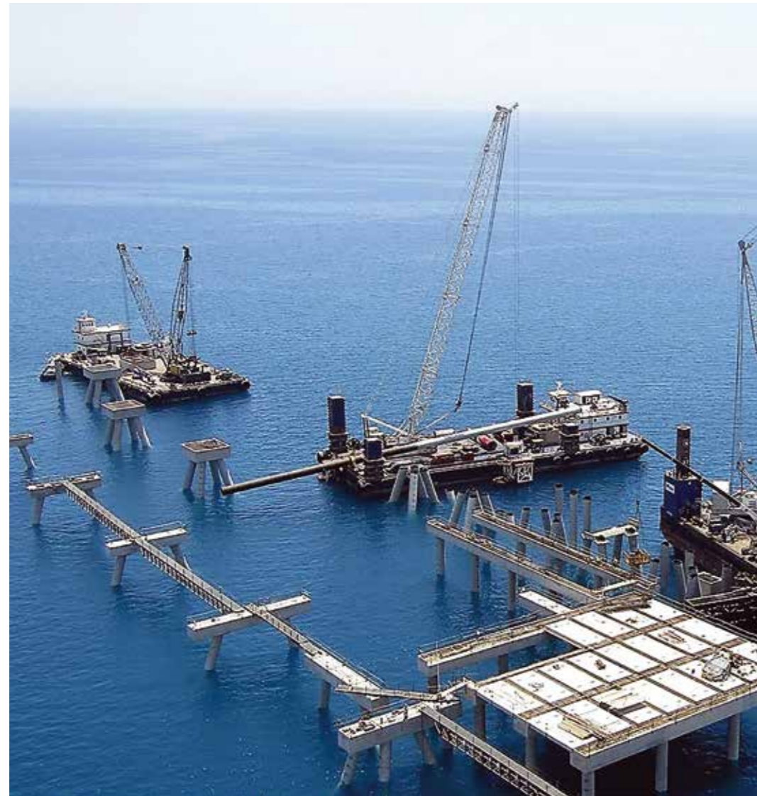
JETTY'S PLATFORM ERECTION
