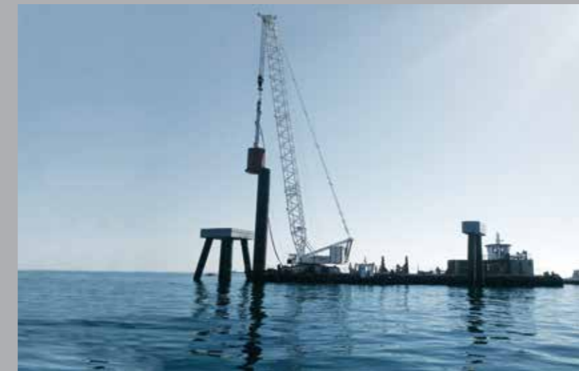
MONOPILES INSTALLATION
