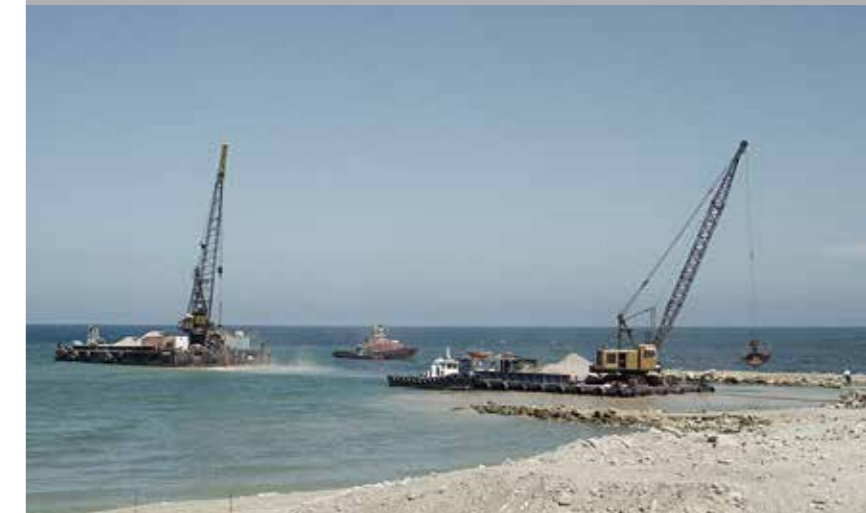
UNDERWATER PIPELINE CONSTRUCTION
