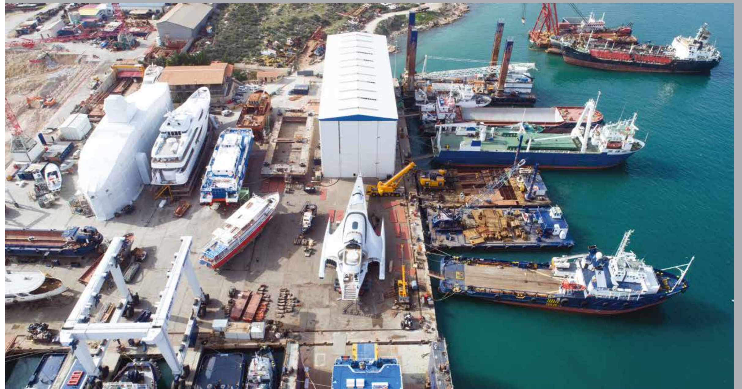
GENERAL VIEW OF COMMERCIAL SHIPYARD IN SALAMINA
